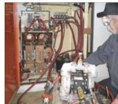
On-site water system clean and flush
