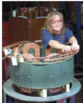
Mold stirring unit overhaul
