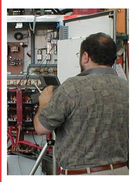
...."Using an infrared imaging camera, a certified engineer can interpret the images to pinpoint problems in your induction system and take proper actions to prevent downtime."
